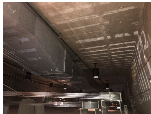
Photo 4- Sprinklers above Stage
