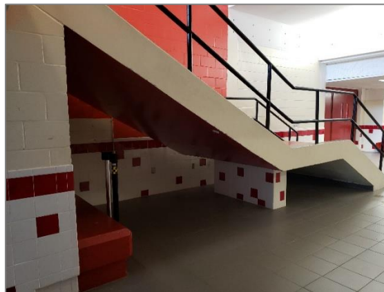
FIGURE 4: STAIR HEADROOM REDUCTION MISSING CANE DETECTION
