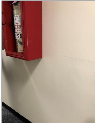
FIGURE 3: FIRE EXTINGUISHER PROJECTION
